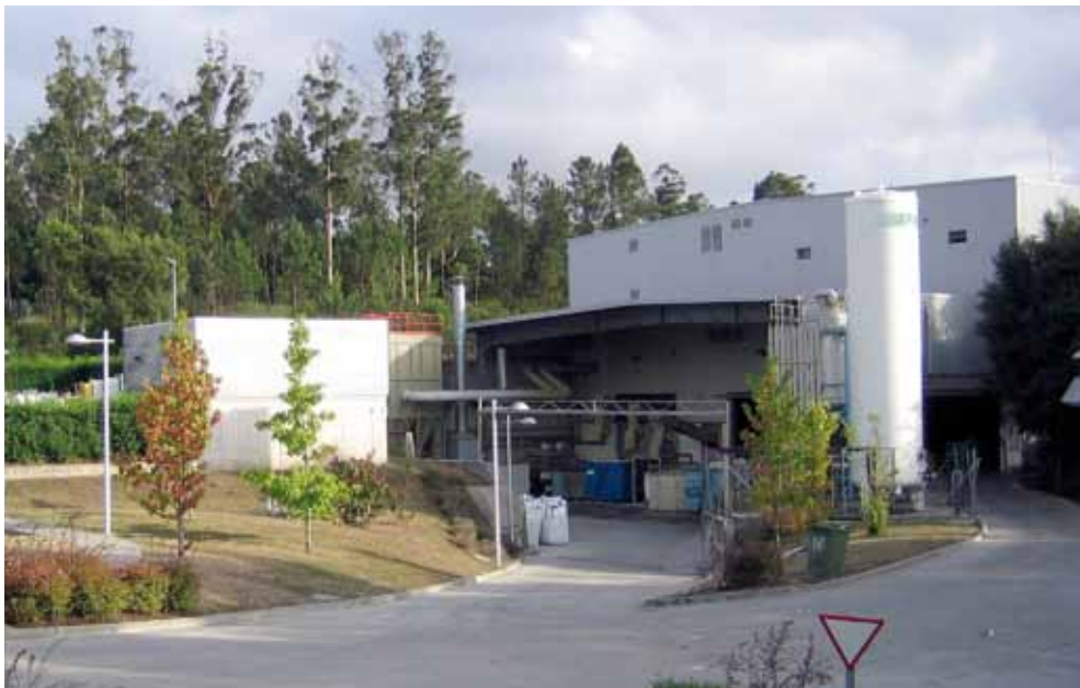
Bulky Waste Treatment Plant Galicia.
